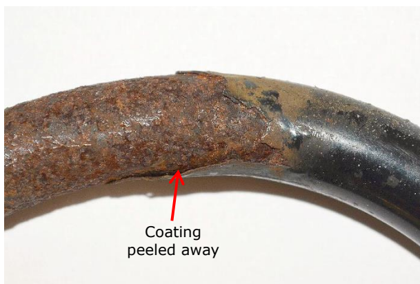
Figure 3. Corrosion progressed along the interface between the coating and the steel.
